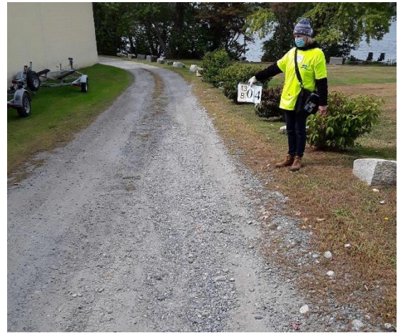
Roads and driveways built to access new development can deliver large quantities of sediment and attached P if not built correctly or maintained properly. (Photo Credit: BLA)
